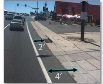
Figure: Gutter Pan Within Bike Lane
